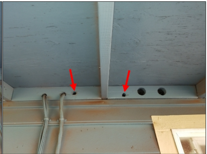
Unplugged holes at eave blocks at left side of the home. (Red)
