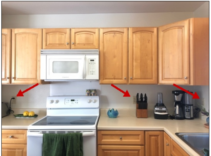
Outlet(s) did not respond to GFI test and does not appear to be GFI protected at kitchen. (Purple)
