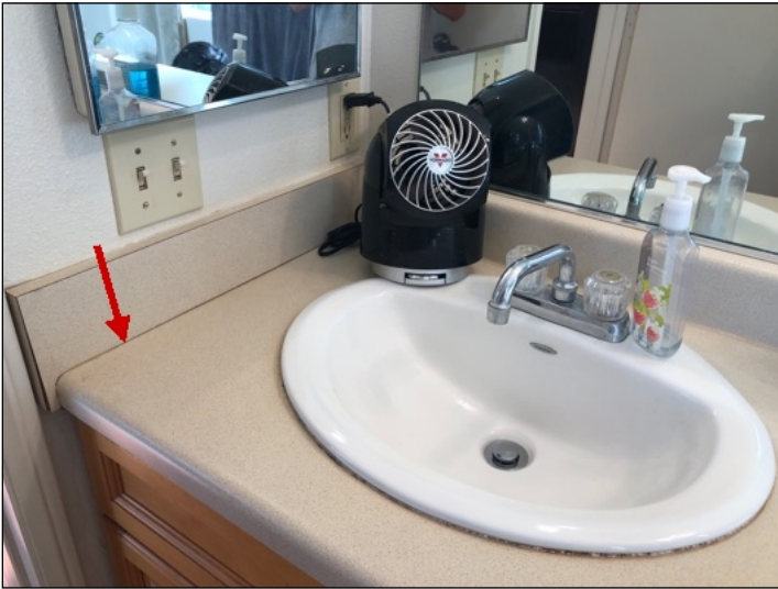
Cracked grout/missing sealant at master bathroom. (Blue)
