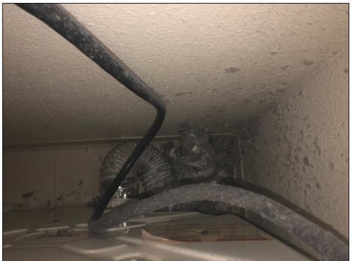
Dryer duct appeared to be damaged or improperly installed. (Red)
