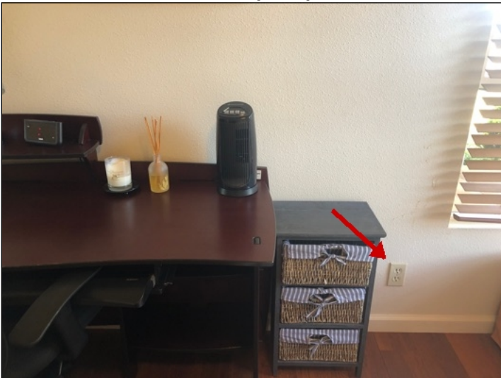
Damaged cover plate at front right bedroom. (Red)
