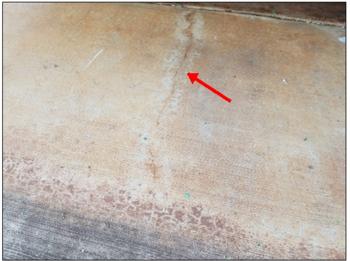
Cosmetic cracks at driveway.
