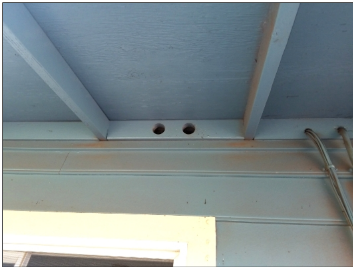
Damaged screens/missing vents at vented eave blocks on left side of home. (Red)
