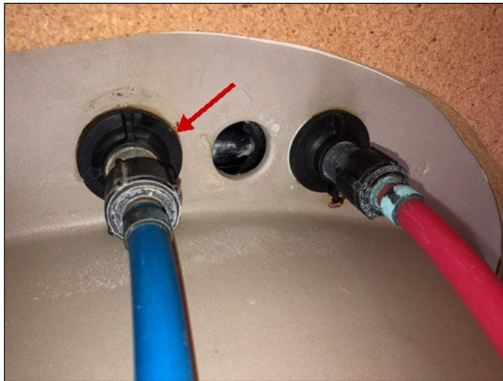
Leak at cold side of plumbing fixture at right hand sink at master bathroom. (Red)
