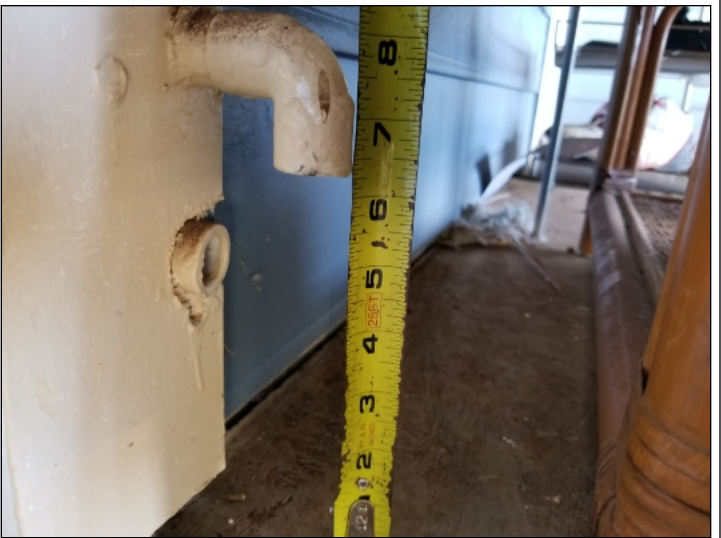
The extension at the water heater relief valve is missing or not the proper length. (Red)
