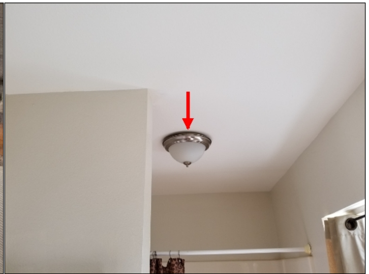
Master bathroom light fixture does not appear secure. (Blue)
