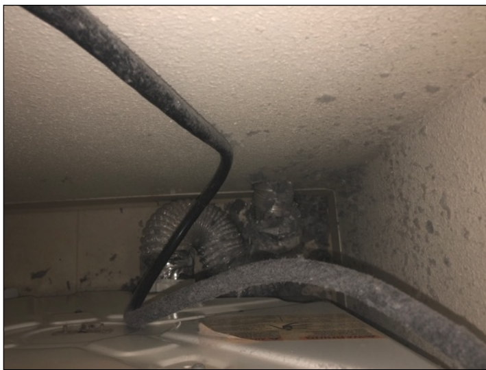
Dryer duct appeared to be damaged or improperly installed. (Red)
