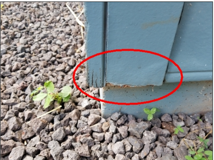
Minor moisture damage at lower sectional is of exterior trim. (Blue)
