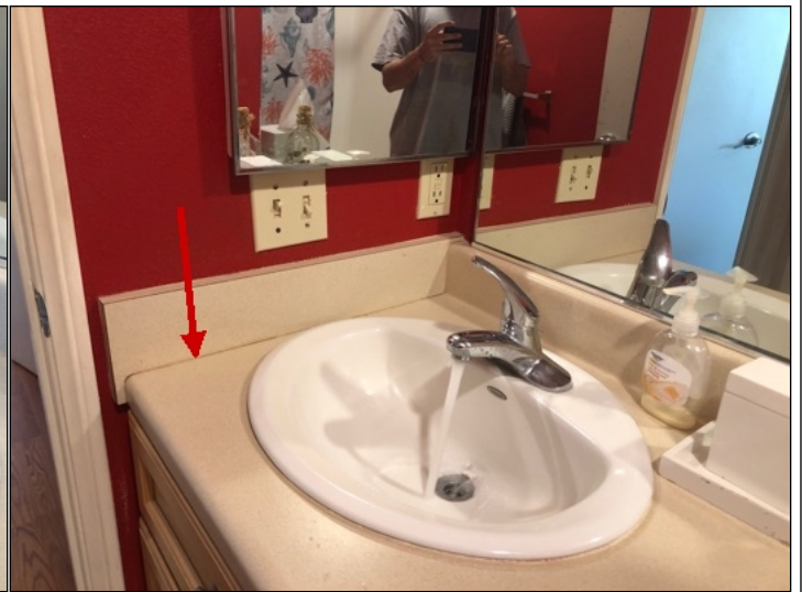
Cracked grout/missing sealant at hallway bathroom. (Blue)
