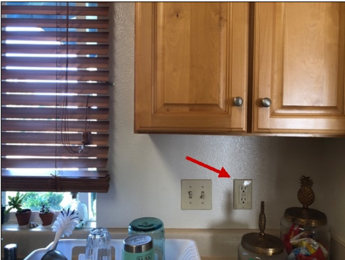
Loose GFI outlet at right side of kitchen sink. (Red)
