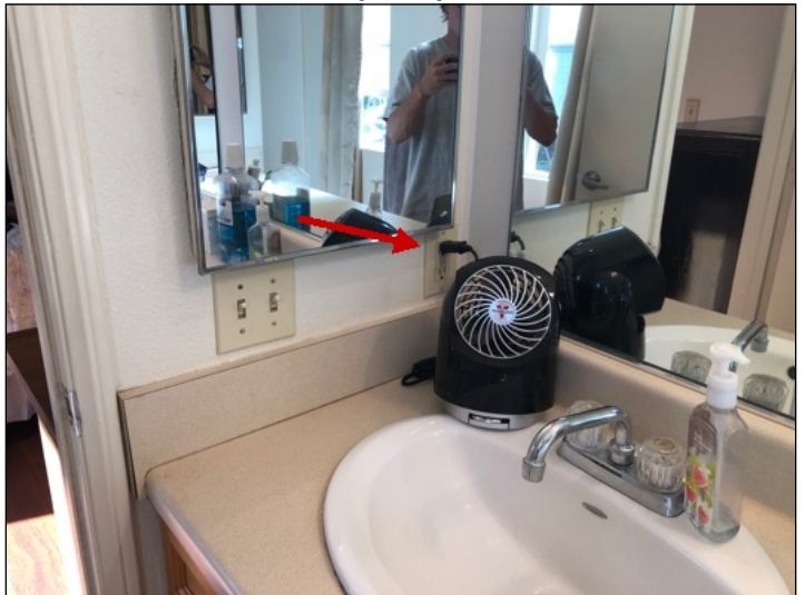
Loose GFI outlet at master bathroom. (Red)
