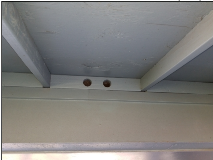
Damaged screens/missing vents at vented eave blocks at right side of carport. (Red)
