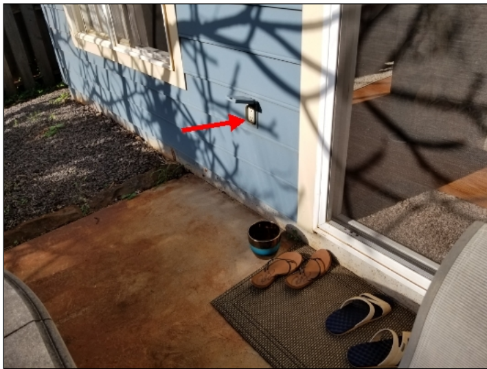
Outlet not functional at rear lanai. (Red)
