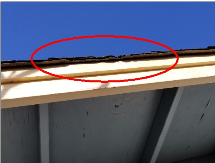
Minor damage to shingle overhang above lanai. Possible damage from nearby tree. (Blue)
