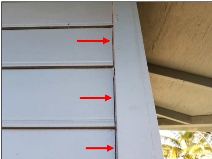
Seal gaps at seams and laps in cladding material. (Blue)
