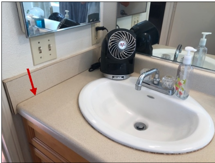
Cracked grout/missing sealant at master bathroom. (Blue)
