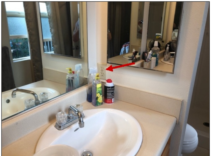
Loose outlet at master bathroom. (Red)
