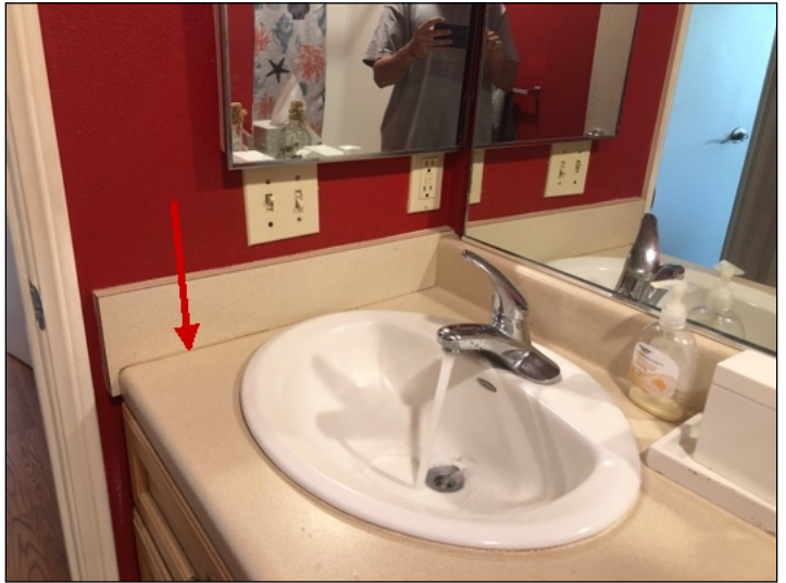
Cracked grout/missing sealant at hallway bathroom. (Blue)
