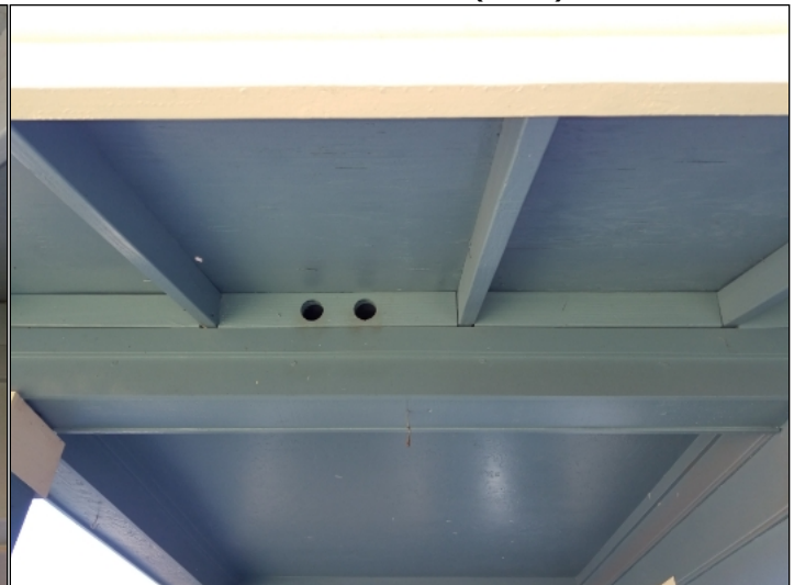
Damaged screens/missing vents at vented eave blocks at right side of front porch. (Red)
