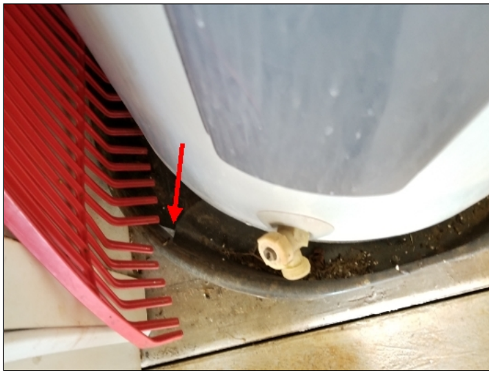
Damaged water heater and the pan. (Red)
