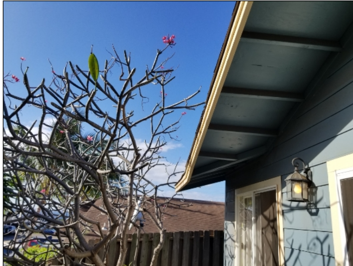
Tree branches were in contact with or near the roof and siding. (Blue)
