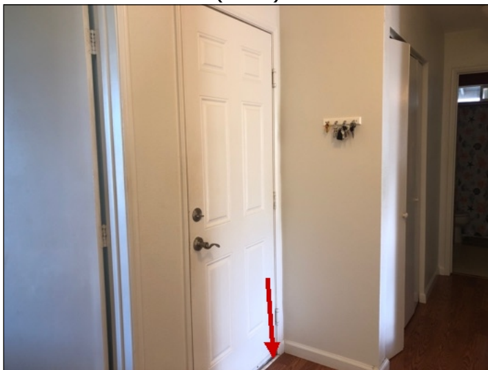
Door(s) rubbed against the jamb or floor, had loose hinges or damaged hardware or otherwise did not operate properly at garage to home door. (Blue)
