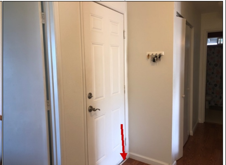
Door(s) rubbed against the jamb or floor, had loose hinges or damaged hardware or otherwise did not operate properly at garage to home door. (Blue)
