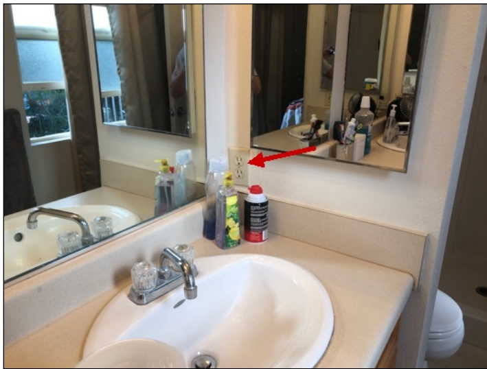
Loose outlet at master bathroom. (Red)
