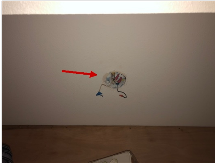
Open junction box at laundry room closet. (Red)
