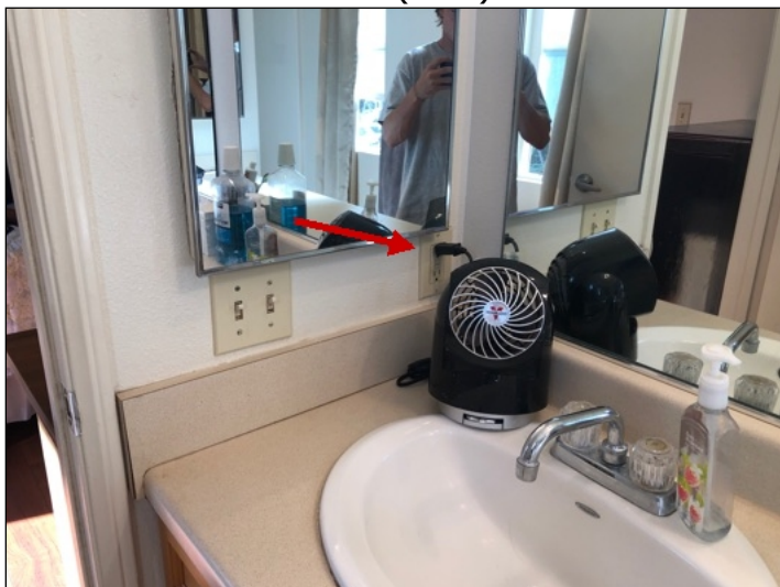
Loose GFI outlet at master bathroom. (Red)
